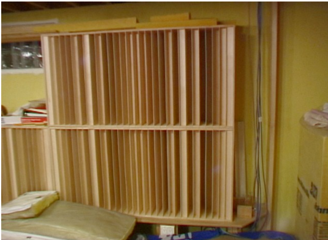
Figure 12. View of part of the mid-range diffusers, prior to fabric covering
